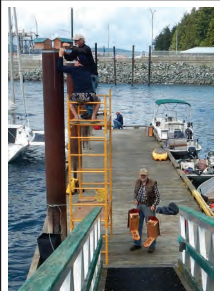
Graeme Johnston, Dave Pick and Peter Karsten installing new martin boxes at the Community Dock May 17, 2020.
