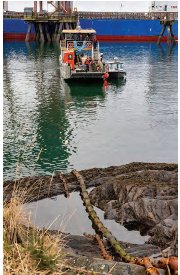
Construction crews working on the Connected Coast connect a subsea fibre line to Ridley Island, outside of Prince Rupert, part of the first 50 kilometres of the build.
