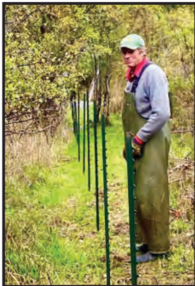
John Mather installing fencing around site.
